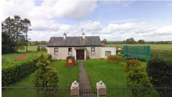
Image of property prior to renovations works commencing
